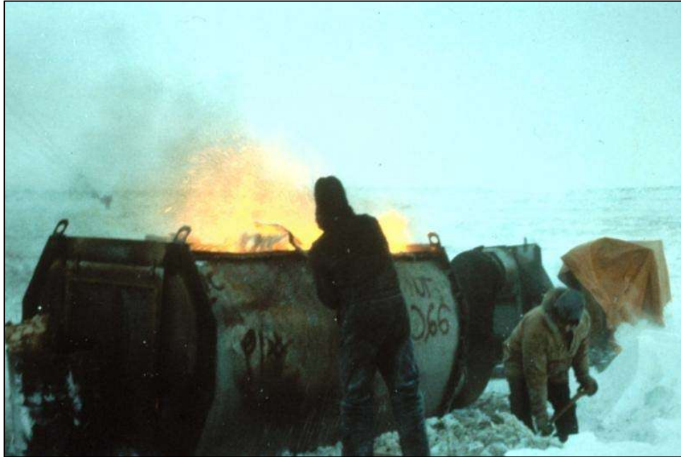
Figure 5-7 Burning oiled snow in a portable air-curtain incinerator. (Source: SL Ross Environmental Research)
