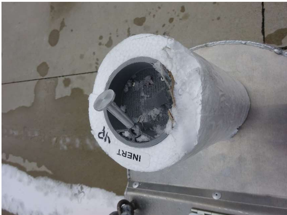
Figure 94. Damage to pin and cartridge
