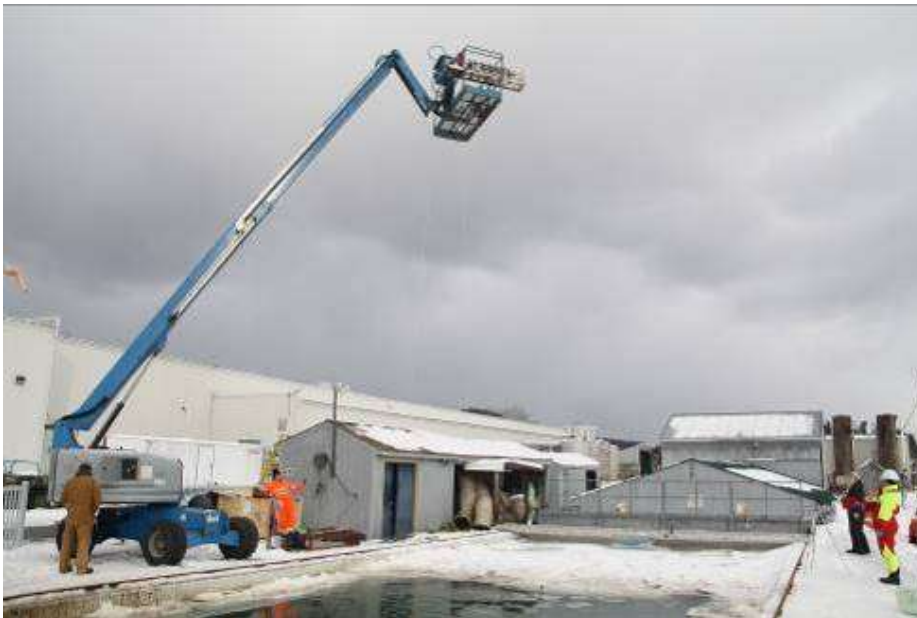
Figure 74 Person Lift Telescoping Crane used to Raise Unit Over GRF Basin
