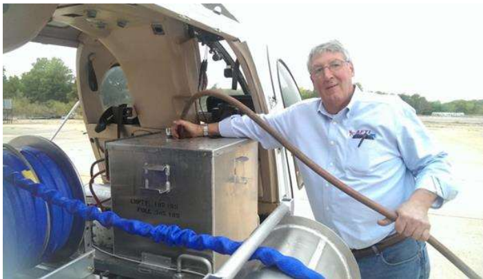
Figure 34: Filling Storage Tank
