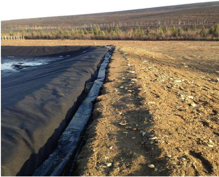
Figure B-4: Keyway Liner and Geofabric Installation
