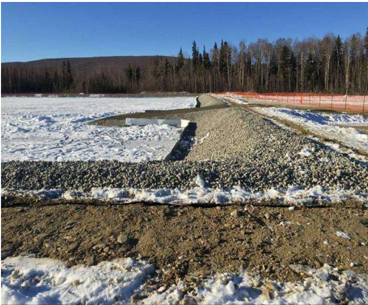
Figure B-9: Rock Armor and flashing installation near the Access Route
