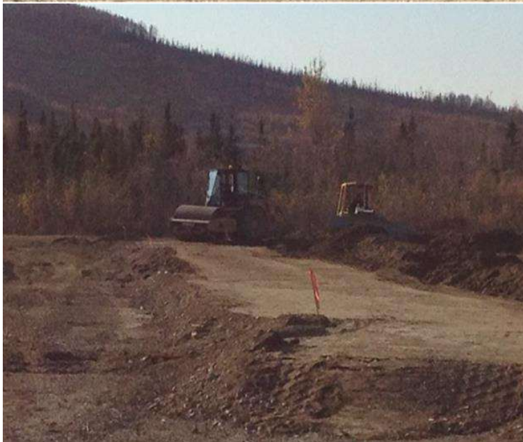
Figure B-3: PFRR Test Basin Berm Grading and Compaction
