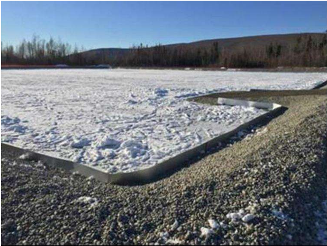
Figure E-5: View of Completed Basin from East Corner Facing West 10/9/14
