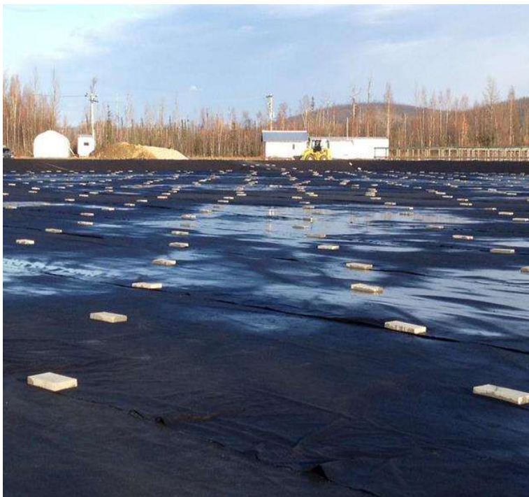
Figure B-6: Concrete Paver placement over Liner/Geofabric
