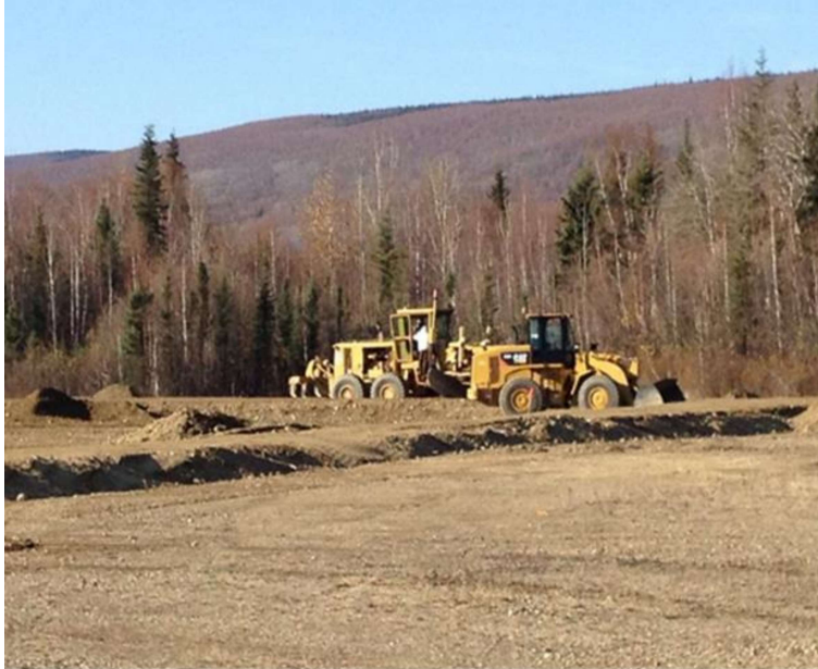
Figure B-2: PFRR Test Basin Site Grading
