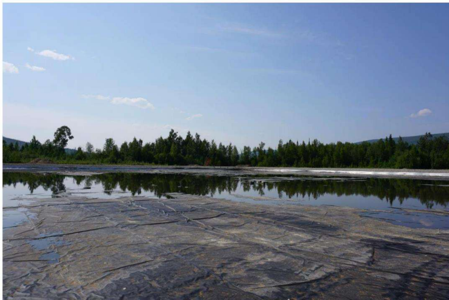
Figure 2: Basin condition on 7/4/15.
