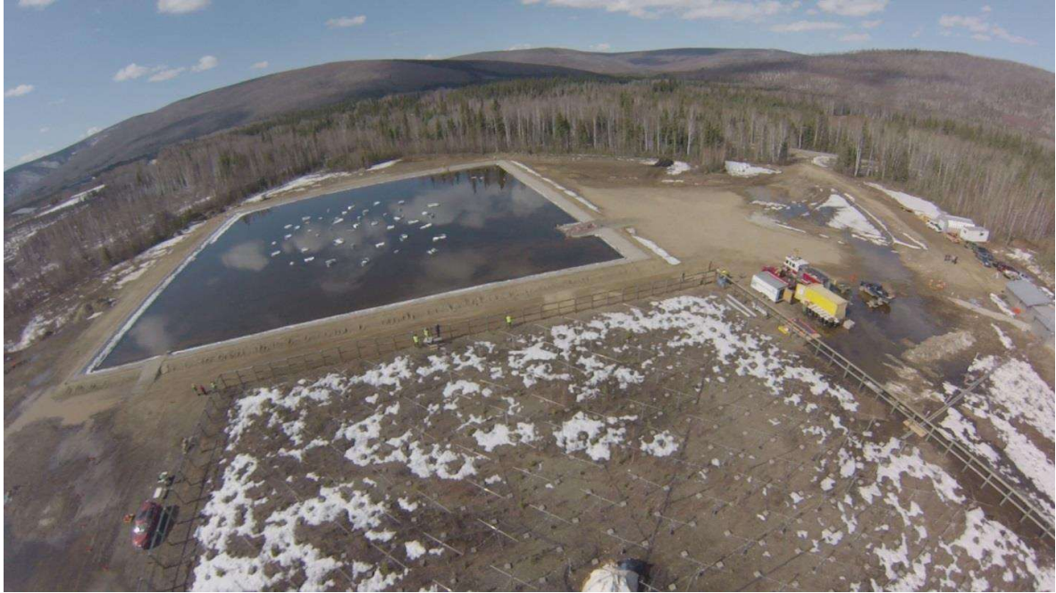
Figure 4: Aerial view of finished basin and site equipment locations
